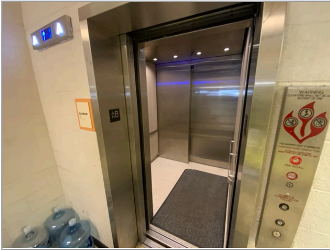
LOBBY LOOKING AT CABS
