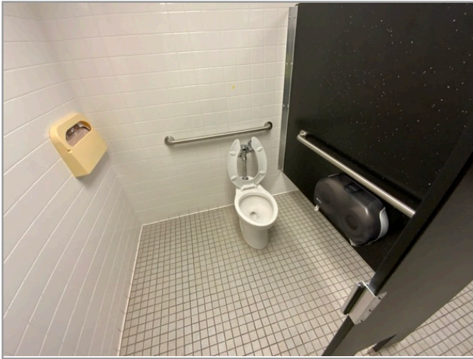
TOILET STALL OVERVIEW
