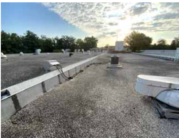
5 - PRIMARY ROOF OVERVIEW
