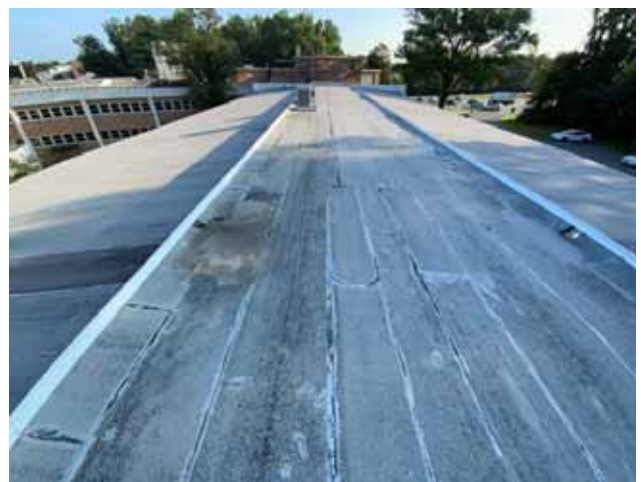
6 - SECONDARY ROOF OVERVIEW
